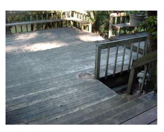
**6. Application:** Before applying Restore-X®, thoroughly wet the surface and broom off excess water. This encourages even penetration of the product. Three important steps to remember when applying Restore-X®: 1) apply a heavy coat using only synthetic brushes or rollers, 2) keep the surface from drying by misting with water\* if necessary, and 3) wait for the product to do the job.
